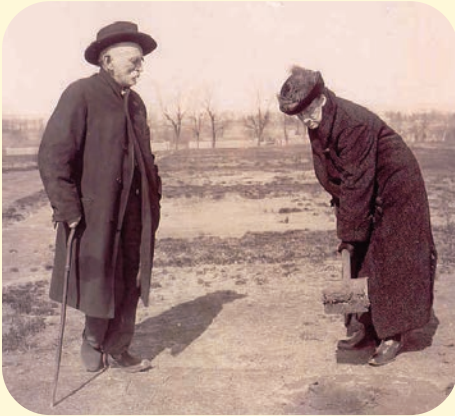
John and Annie Warner breaking ground for Gettysburg Hospital
